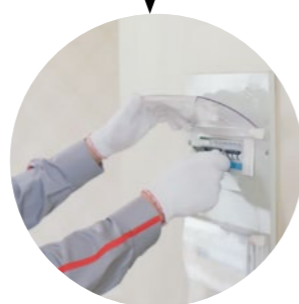
Light electrical repair
