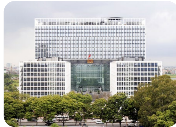
Maintain the optical cable system of the Ministry of Public Security
