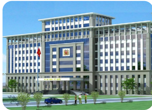
Package maintenance of 530 air conditioners at Tra Vinh Provincial Police Headquarters
