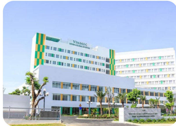
Maintain the water heater system at Vinmec Danang Hospital
