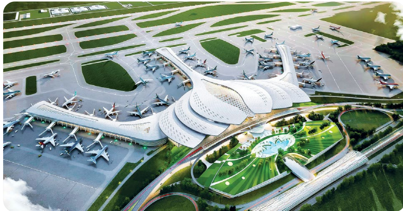
LONG THANH AIRPORT PROJECT Investor: Vietnam Airlines Corporation (ACV)
