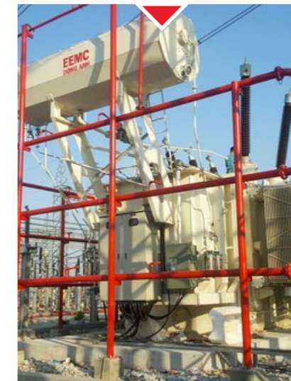
INFRASTRUCTURE OPERATION OF 220KV BAC NINH SUPPLY STATION 3 Investor: Song Da Corporation
