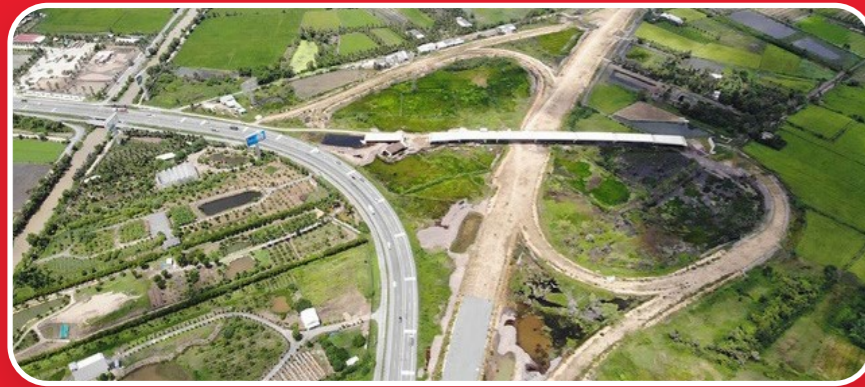
TIEN GIANG CAI BE INTERCHANGE CONSTRUCTION PROJECT Investor: Ministry of Transport
