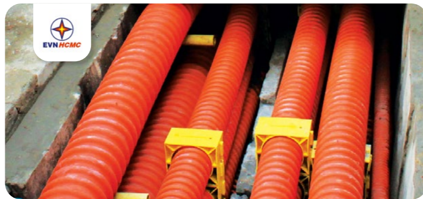
EVN HCMC underground construction project
