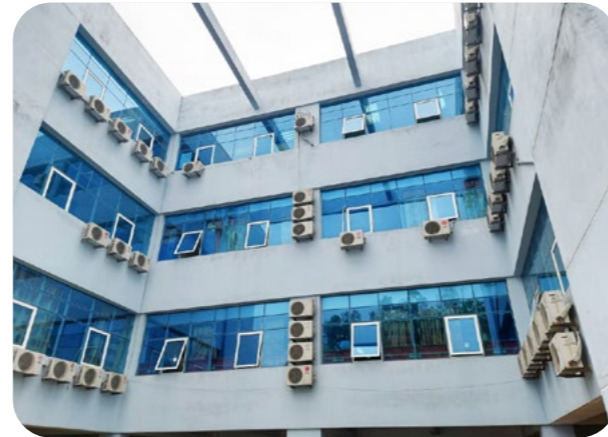
Maintenance of air conditioning system at Bac Kan Provincial General Hospital
