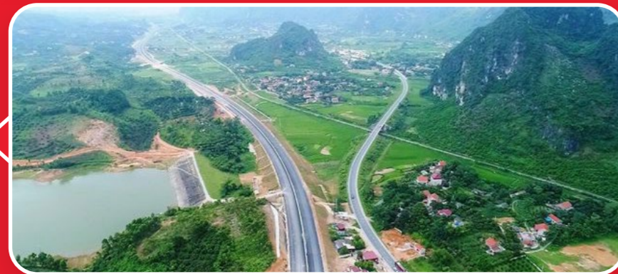
BAC GIANG - LANG SON EXPRESS BRIDGE CONSTRUCTION Investor: Ministry of Transport
