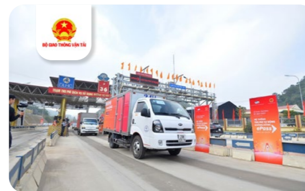
Non-stop toll station project EPASS
